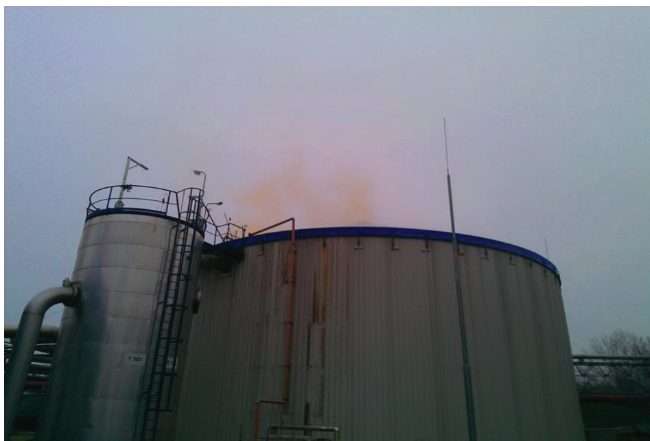
Figure 4 Evidence of nitrous gases including NO 2 rising from the denitrification reactor.
