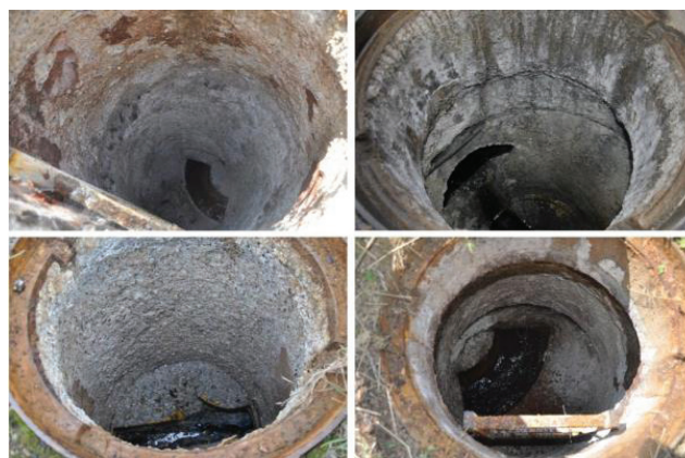
Figure 2 Concrete degraded by biogenic acids in the sewer system [17].
