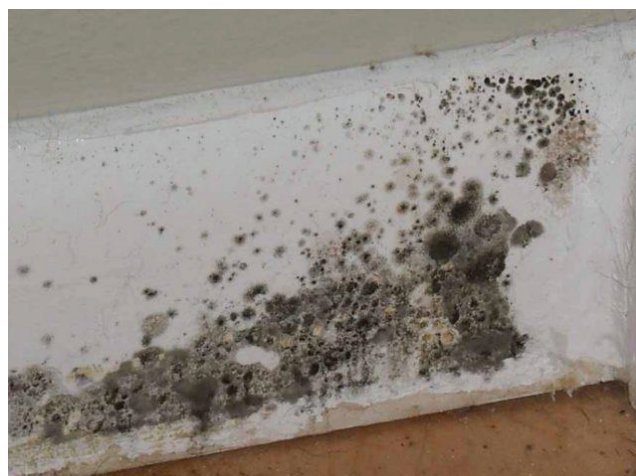
Figure 5 Concrete infested with Stachybotrys chartarum [31].
