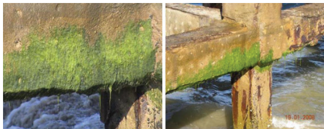
Figure 4 Ulva Fasciata seaweed growth on concrete [26].
